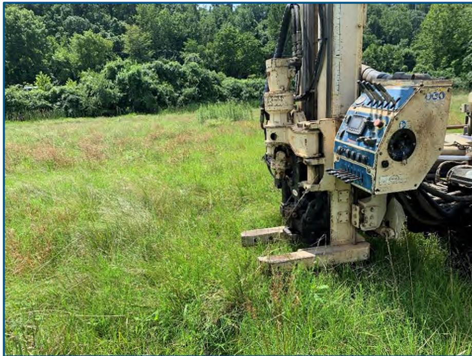
Photograph # 2 Facing south, looking at the SS-3/SB-3/GW-3 location.
