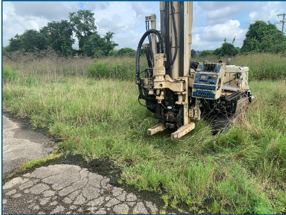
Photograph # 5 Facing northwest, looking at the SB-7 location.
